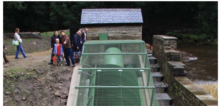
The archimedean screw in motion.
