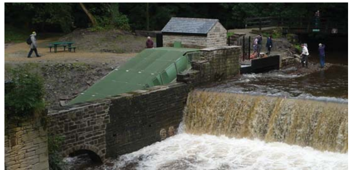
Torrs Hydro New Mills
